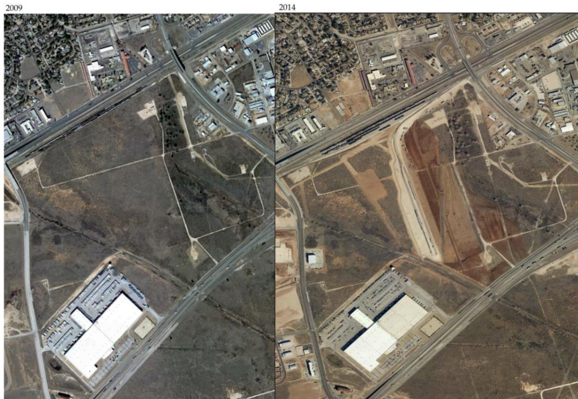
Figure 9.6 Union Pacific Odessa Rail Yard & UPDS Railport
